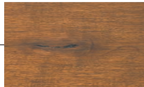
Surface holes and hairline cracks
